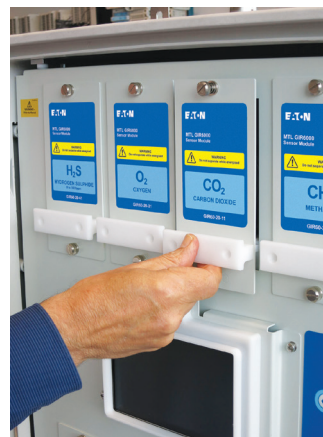
Figure 7.2 - Module replacement
